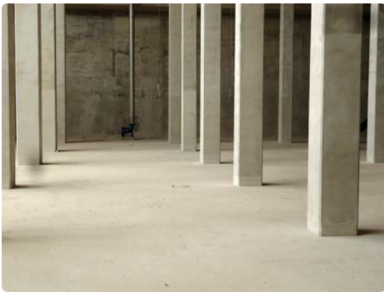
Above and bottom left: The interior of the SBR plant comprises a network of tall, slim, 500–600mm square columns.
