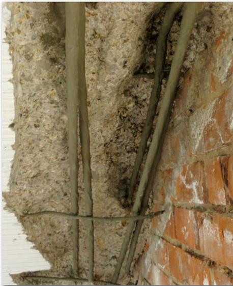
Cut back to steel reinforcements
