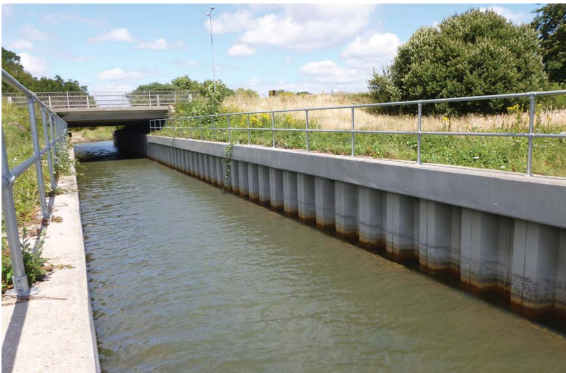
Left: Project at Creekmoor, Poole after application of cementitious coating.
