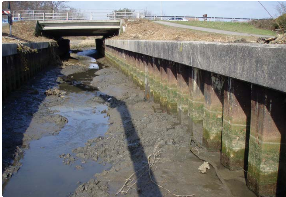
Above: Project at Creekmoor, Poole before application of cementitious coating.
