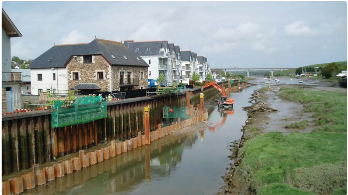
Right: Wadebridge Estuary in Cornwall. Below: Application of coating.
