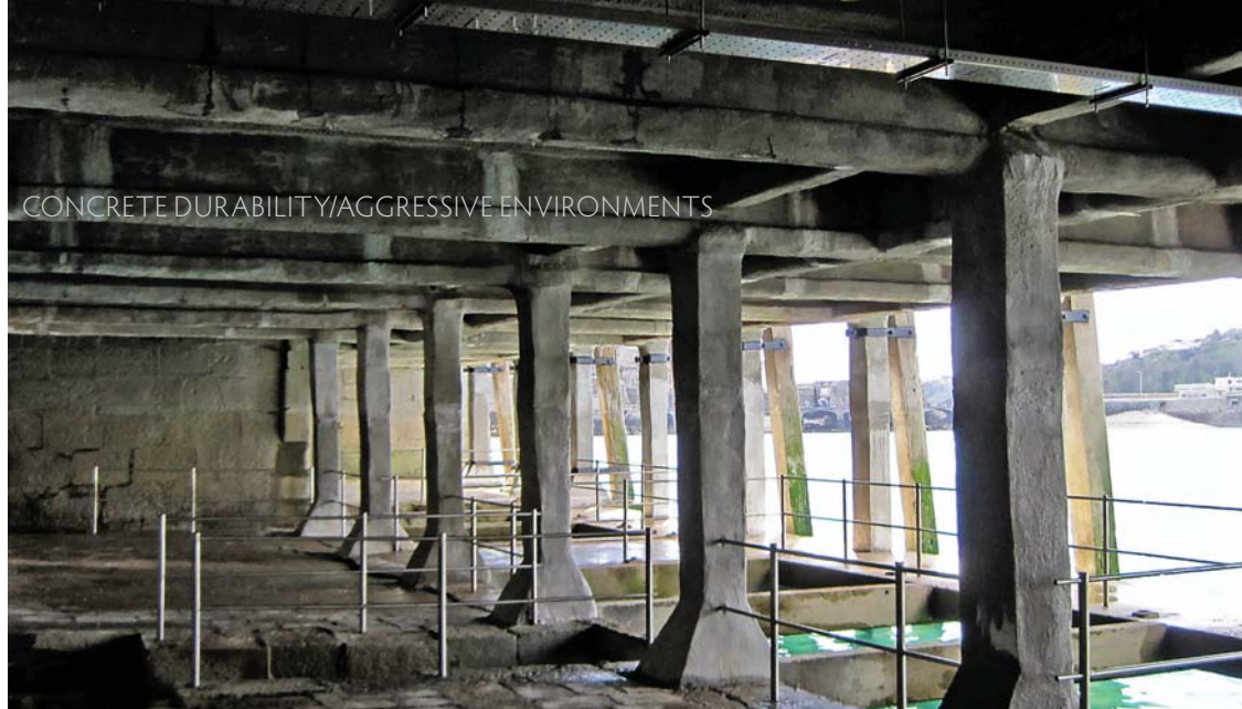
Cementitious coating has been applied at St Peter Port Docks.
