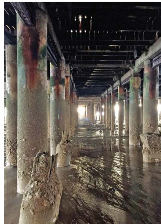
The extent of chloride attack to the reinforced beams and columns at Clacton Pier.
