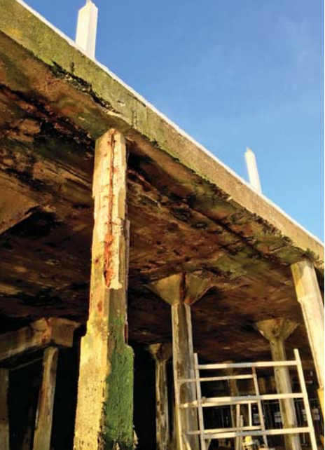
Chloride attack to the reinforced beams and columns at Clacton Pier.
