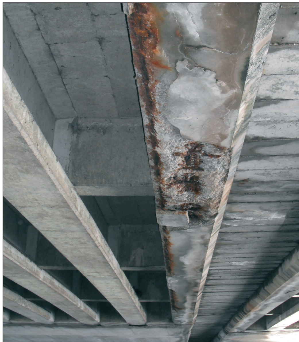
Chloride-affected concrete and a typical application for Cementitious Coating 851.
