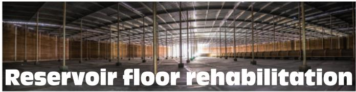
Over 73 tonnes of a high performance cementitious coating manufactured by UK-based Flexcrete Technologies Limited. one of the AkzoNobel group of companies, has been delivered by air freight to Sydney to meet the special requirements of a major floor rehabilitation project at an 86ML potable water reservoir in the Newcastle region of Australia.
