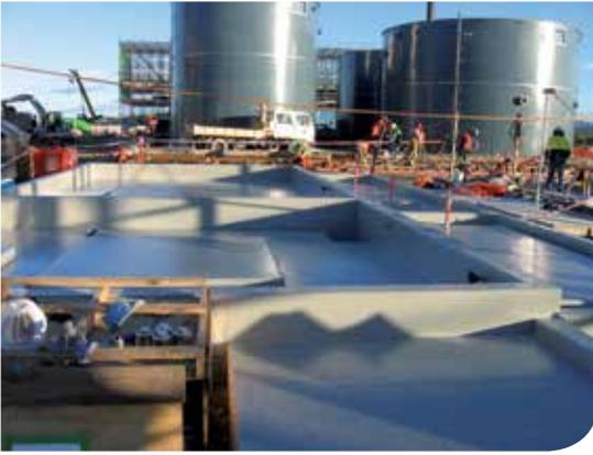
the application of a chemically resistant top coat within one more week. By adopting this approach, the normal 28 day cure period for freshly cast concrete can be waived, thus saving valuable time. Cemprotec E942 is certified to EN 1504-2 for Protection against Ingress and is in use worldwide.
