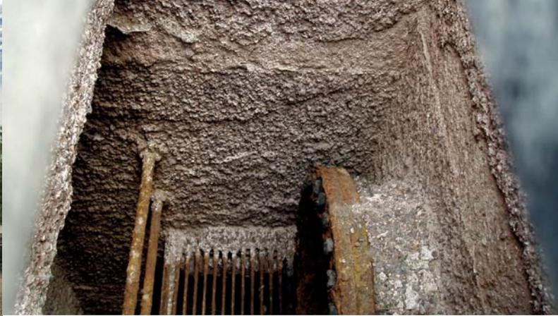
Concrete deterioration caused by sulfuric acid attack.
