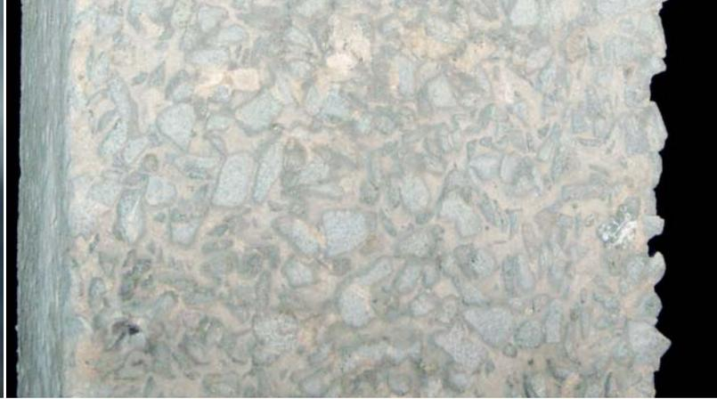
Typical soft water damage to a concrete column in a service reservoir.
