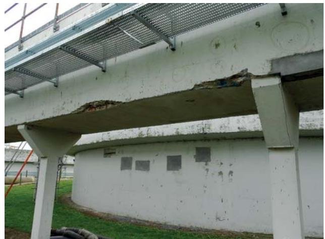
Example of concrete deterioration to inlet channels.
