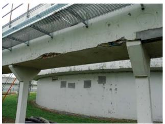
Example of concrete deterioration to inlet channels.
