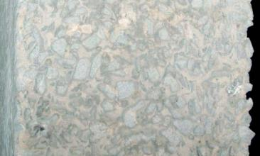
Typical soft water damage to a concrete column in a service reservoir.
