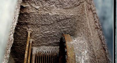
Concrete deterioration caused by sulfuric acid attack
