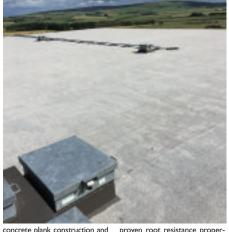
concrete plank construction and considerable movement was expected. As a result, Fraser Bruce Group proposed the reinforcement of the Cemprotec Elastic with Cemprotec Geo80, a thermally bonded non-woven geotextile, to give increased toughness to the coating and enhanced crack bridging proper-Over formed joints. Cemprotec 2000-S, an elastomeric. breathable polyurethane based reinforcing tape, can be used to provide effective waterproofing in these critical areas.
