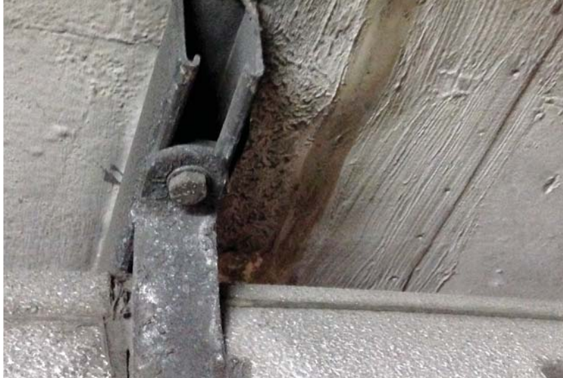
The expansion joints in the access tunnel had previously been waterproofed with a Hypalon over-bandage system adhered with an epoxy resin.
