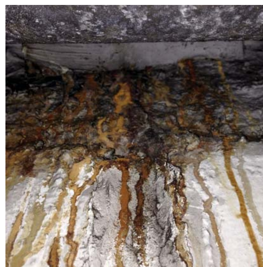
Rusting and exposure of steel reinforcement.
