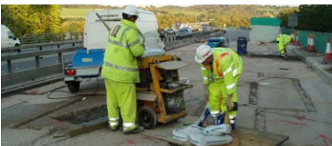
Fastfill sets in just 10 minutes & can achieve a final strength of over 60MPa.
