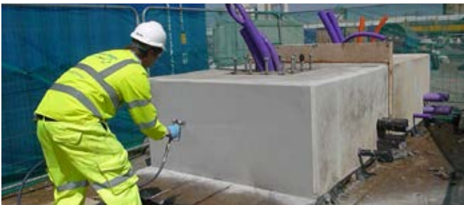
Cementitious Coating 851 effectively reinstates cover & protects from chlorides.
