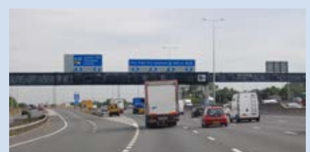
Flexcrete's repair & protection solutions are ideal for use on SMART motorway construction.
