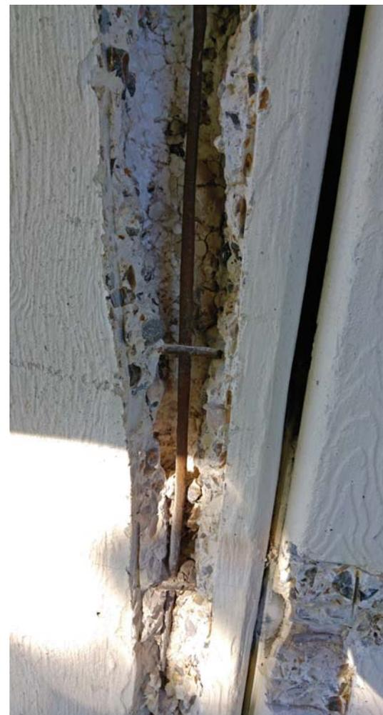
The concrete cut back to the steel reinforcement.
