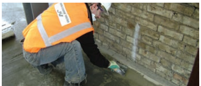
Monolevel RM is fibre-reinforced for added strength and durability.
