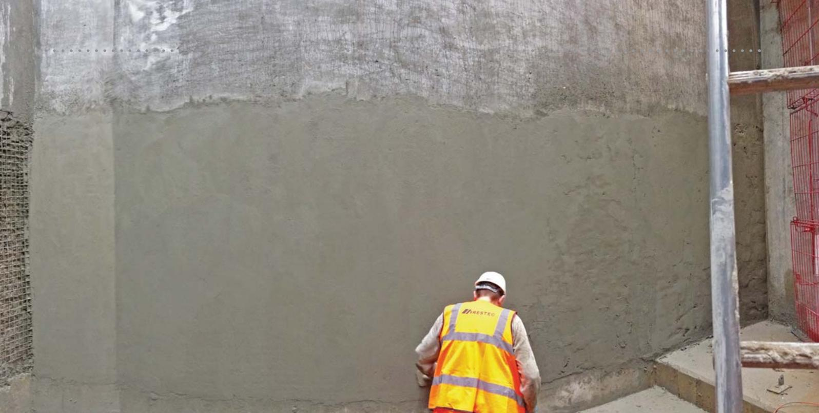
*Due to its very low rebound properties, Monomix WS can be easily applied in enclosed locations.*
