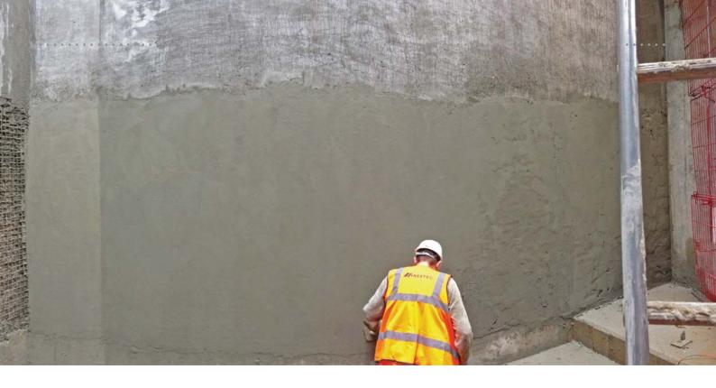
$\label{thm:condition} \textit{Due to its very low rebound properties, Monomix WS can be easily applied in enclosed locations.}$
