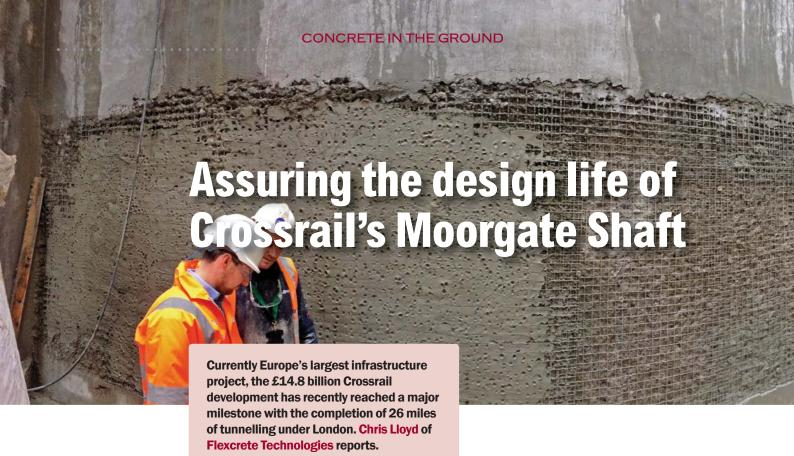
An area of 50m2 was reinstated on the new concrete shaft walls. assuring a 120-year design
