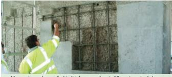
Monomix can be applied in thicknesses of up to 80mm in a single layer.
